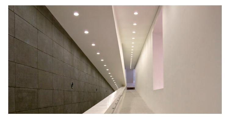
OKT LED commercial downlights have been upgraded 4th generation since 2013. This 4" commercial LED downlight is powered by high efficiency external LED driver, which continuous dims to 10% that works with many types of controls. It has CCT selectable and wattage adjustable functions to maximize light compatibility by dip switch. Spun aluminum reflector integrated with haze finish and white trim ring with shadow free. Deeply regressed diffusing lens conceals the LEDs from direct view.
